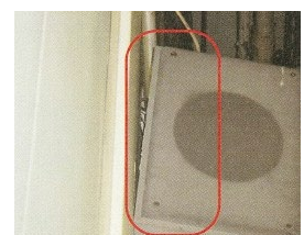
拡声装置の取付不良❖ 3
